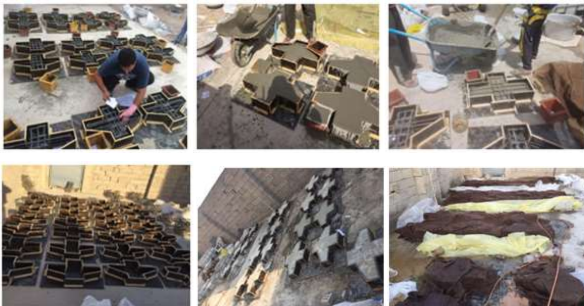
Figure (4) Casting and Curing of R.C. corbels
