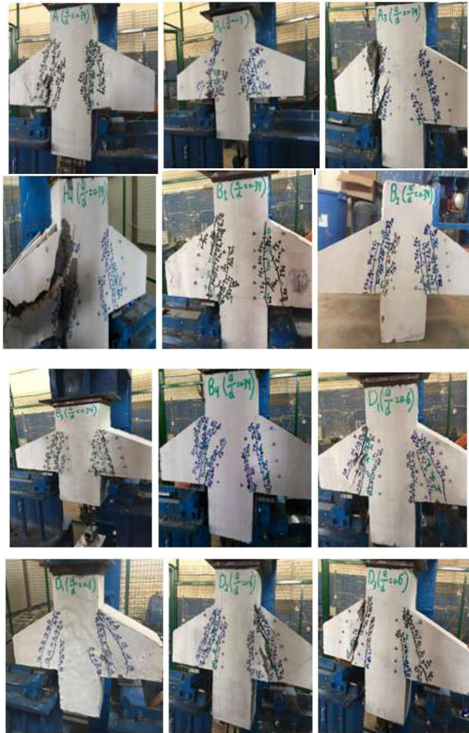
Figure (9) Cracks Pattern of Corbels
