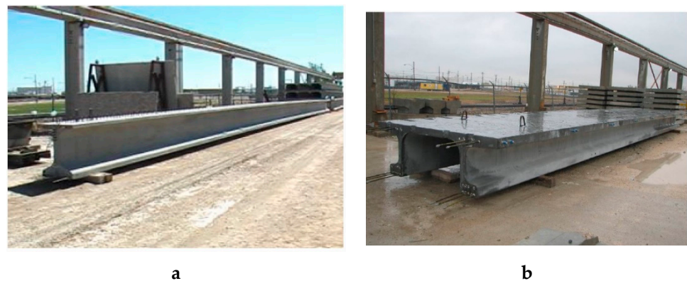
Figure 5. Representative apps of UHPCs in BEs: (a) I-formed girder [115]; (b) Pi-formed girder [116].
