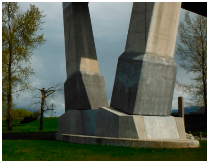
Figure 4. Representative apps of UHPC in BEs: pier jacket [99].
