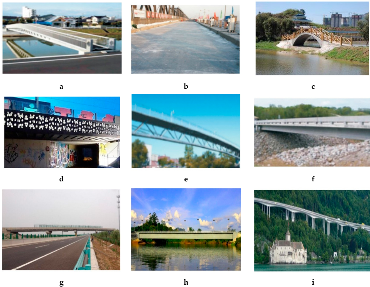
Figure 3. Typical apps of UHPC in BE: (a) Sakata-Mirar foot BE; (b) Zhaoqing Mafang BE; (c) ultra-high-performance, fiber-reinforced concrete arch BE in Fuzhou University campus viaducts; (d) Martinet foot BE; (e) Sherbrooke pedestrian BE; (f) Mars Hill BE; (g) Shijiazhuang to Cixian highway BE; (h) Batu 6 BE; (i) Chillon [53,91–94].
