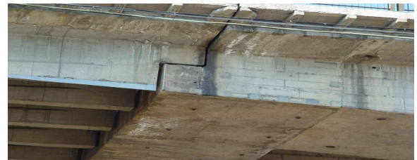
Fig. 10 Hanging beams in the part of corbel
