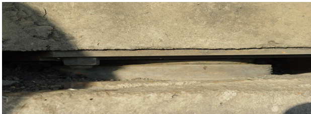
Fig. 9 Bearings of corbel
