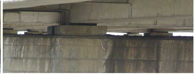
Fig. 8 Bearing of simply supported T-beams
