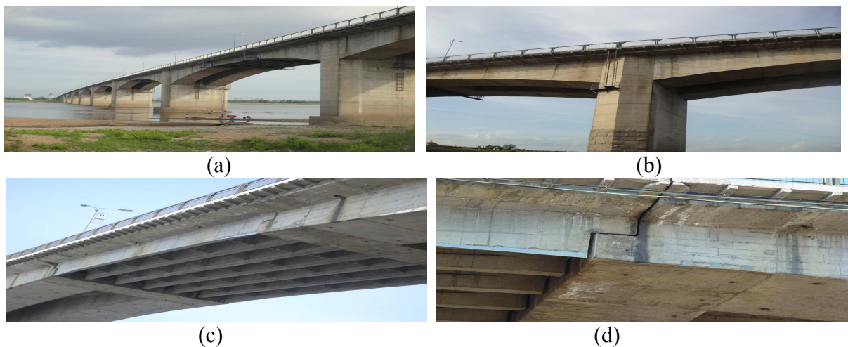
Fig. 1 View of bridge structure: (a) Spans of bridge view, (b) T-shape structure, (c) Hanging beam between two T-shape structure, (d) Corbel view
