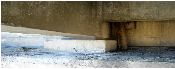
Fig. 7 Bearings of approach supports
