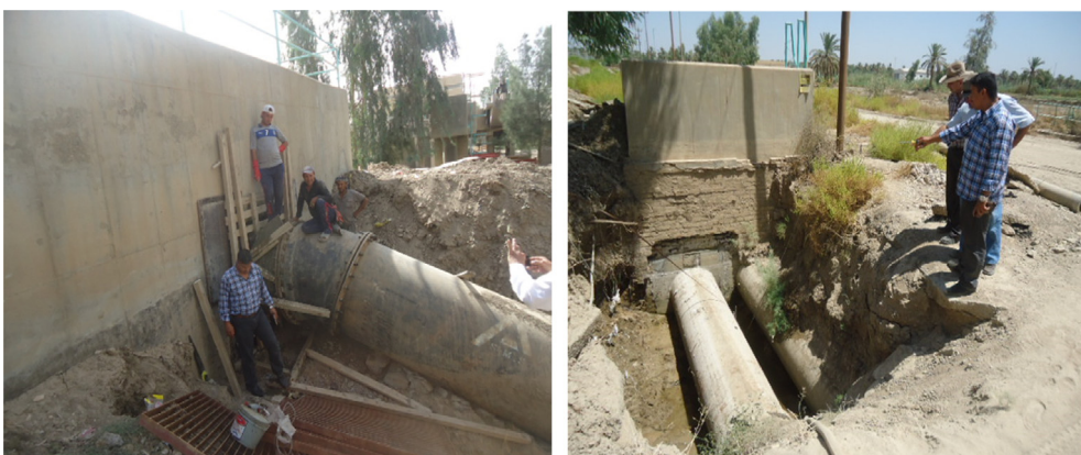
Fig. 5. Connection area left uncover for long time inspection.
