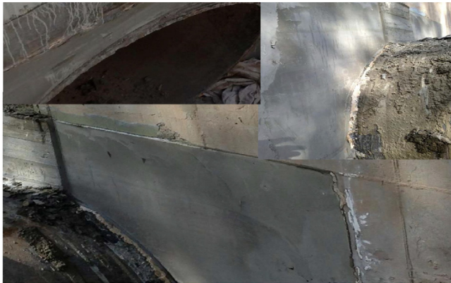
Fig. 4. Final surface around the connection area.
