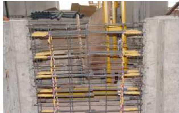
Fig.3 The strain gage layout of shear-key
