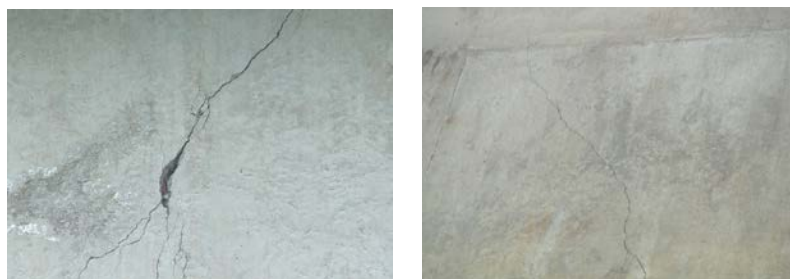
Fig. 2: The cracks in the box girders; (a) outside of box girder, (b) inside of box girder
