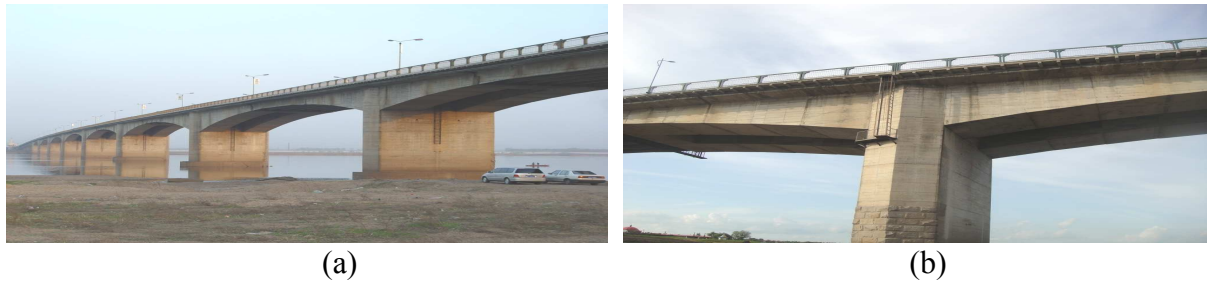
Fig. 1 View of a bridge structure: (a) spans of bridge view, (b) T-shape structure
