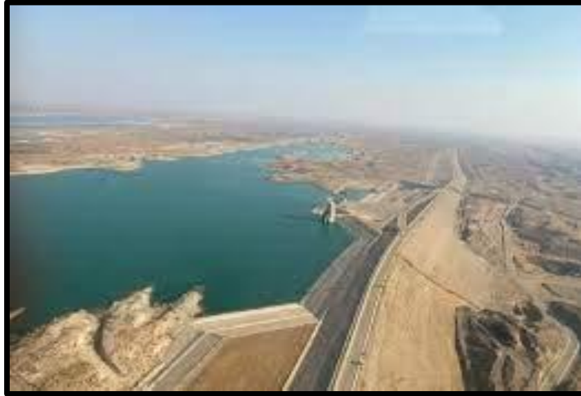
FIGURE 4. Al-Adhaim dam shape
