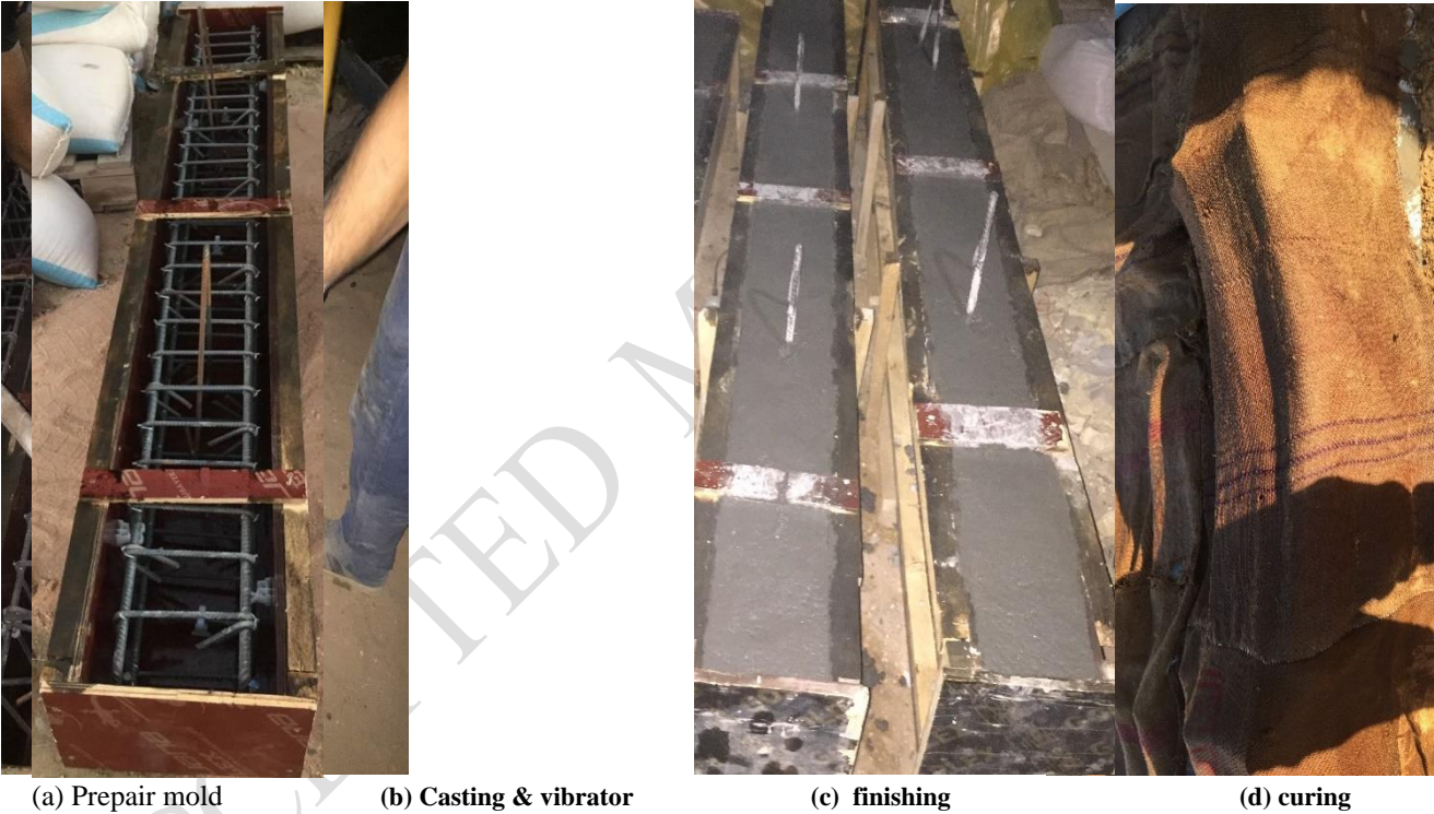
Figure 4. Preparing mold and casting Specimens
