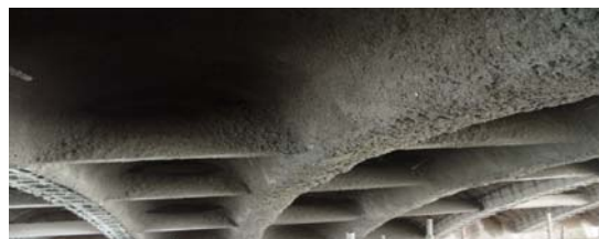
Figure 14: The first layer of sprayed concrete
