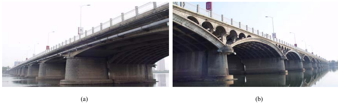
Figure 1: Jilin highway double-curved arch concrete bridge (a) side view of the old simply supported beam bridge, (b) side view of the new arch bridge
