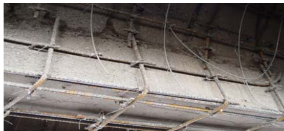
Figure12: Planting steel bars in arch rib
