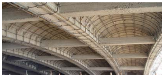
Figure11: Planting steel bars in arch rings
