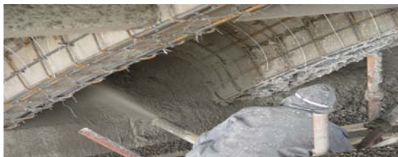
Figure13: Spraying the concrete
