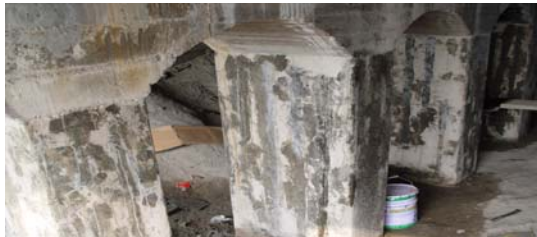
Figure 15: Repair the piers of spandrel arch
