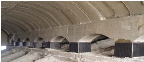
Figure 17: Spandrel arch piers strengthening
