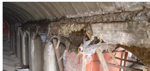
Figure 18: Pier cap repair
