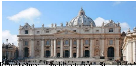
(Renaissance architecture) St. Peter's Church (Vatican) in Rome for Architects Bramante and Michelangelo, in 1450, then Architect Bernini added two sides to it https://en.wikipedia.org/wiki/St._Peter%27s_Basilica#/media/File:Rome_San_Pietro.jpg Figure 7b :Architectural additions before the Industrial
