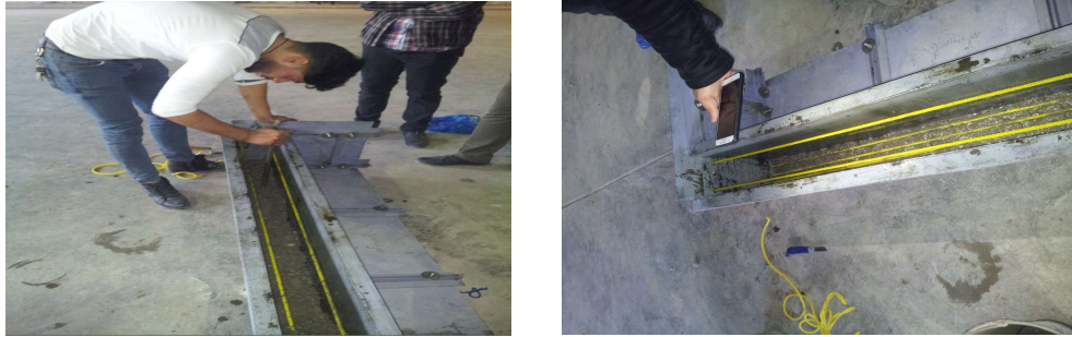
Plate 1. Steel mold used and concrete casting process.
