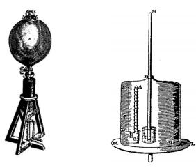
Fig. 4. Designed Piston vacuum pump from 1658 to 1659 by Robert Boyle and Robert Hooke.
